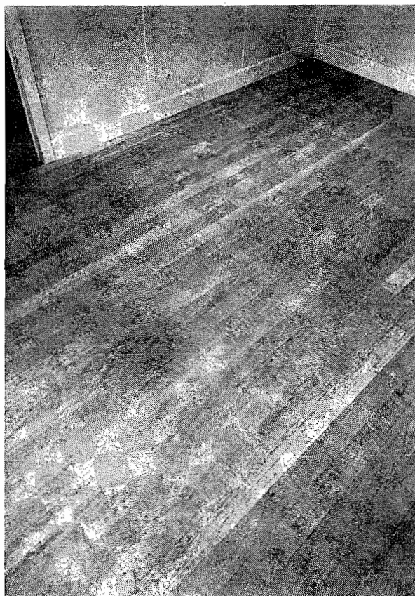
Fig. 2. General view of Red Gum floor after laying but prior to sanding or finishing. The section nearest the door shows "select" grade material, and that nearest the farthest wall shows standard grade.
